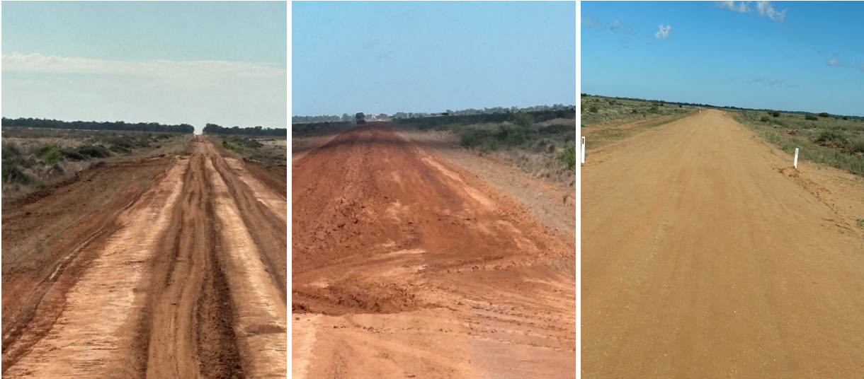
Booligal Gunbar Road maintenance grade
