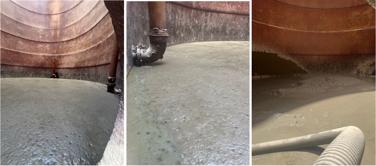
Leonard St raw water reservoir cleaning - Before
