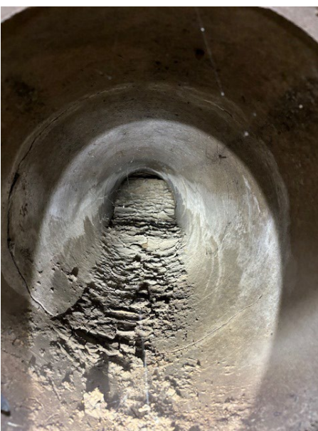
Stormwater before cleaning
